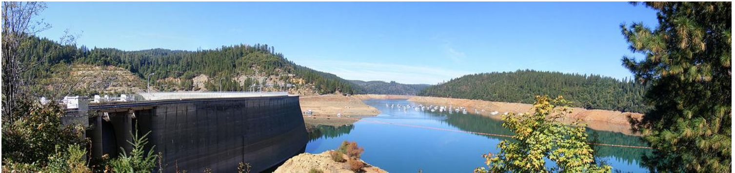
New Bullards Bar Dam and Reservoir, © Justin Smith / Wikimedia Commons, CC-BY-SA-3.0 (see References section)
